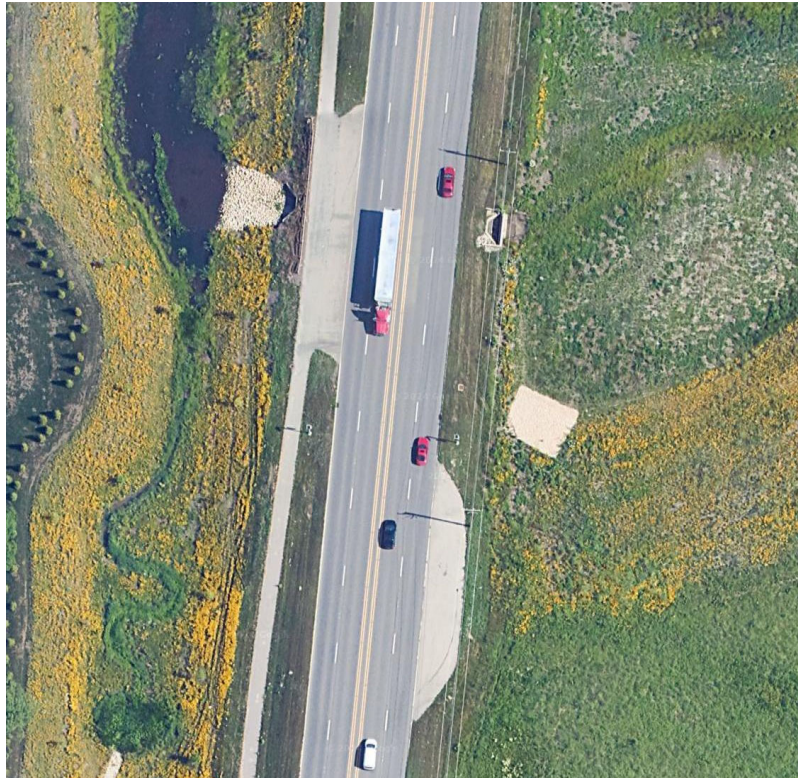
Figure 6-6. Truck Pullouts in Kane County, IL
