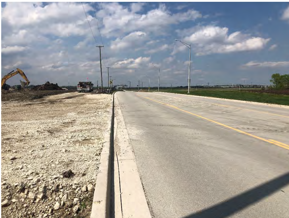
Figure 6: The stabilized entrance is in good condition and no tracking was observed along McLinden Road; view to north.
