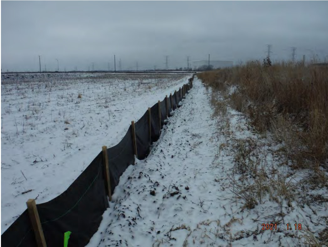
Figure 5: Silt fence in good condition along south perimeter of Site; view to east.
