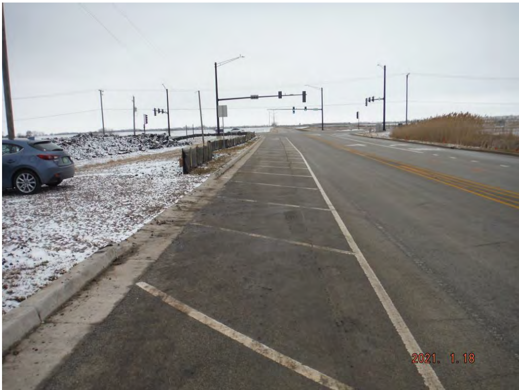
Figure 2: No tracking of sediment and debris observed at east entrance of Site; view to north.
