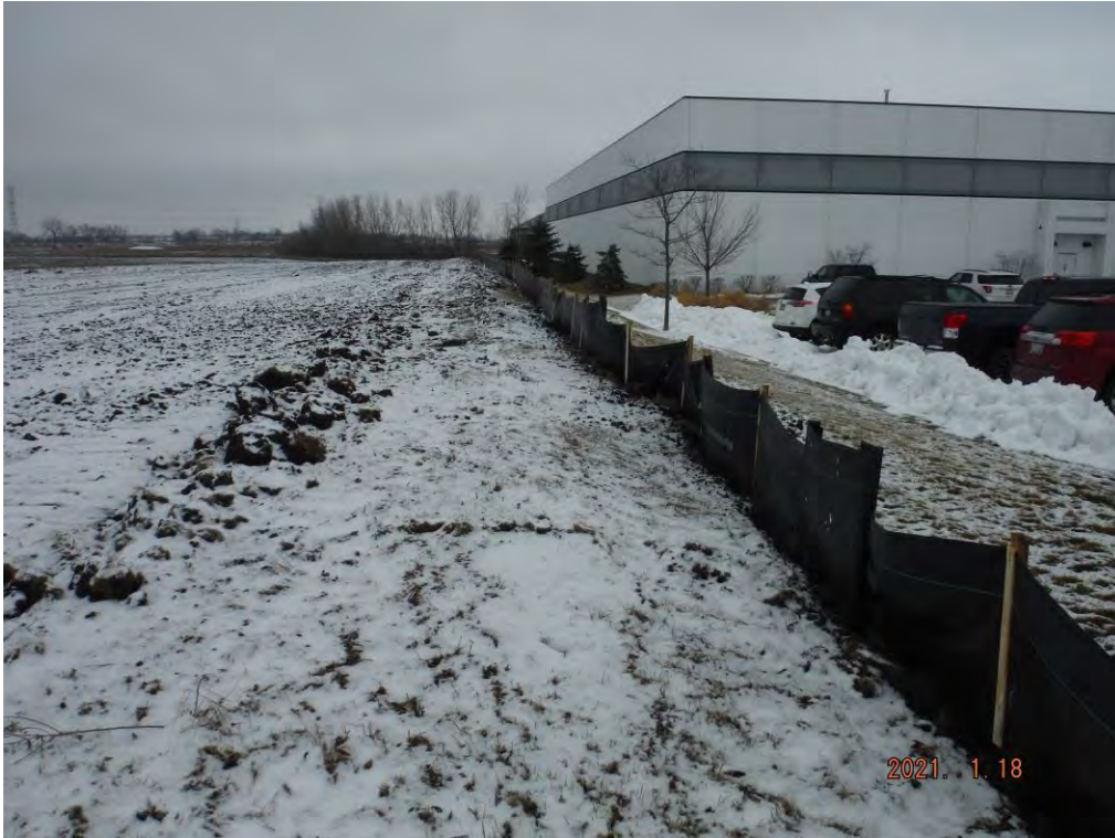
Figure 3: Silt fence in good condition along west perimeter of Site; view to south.
